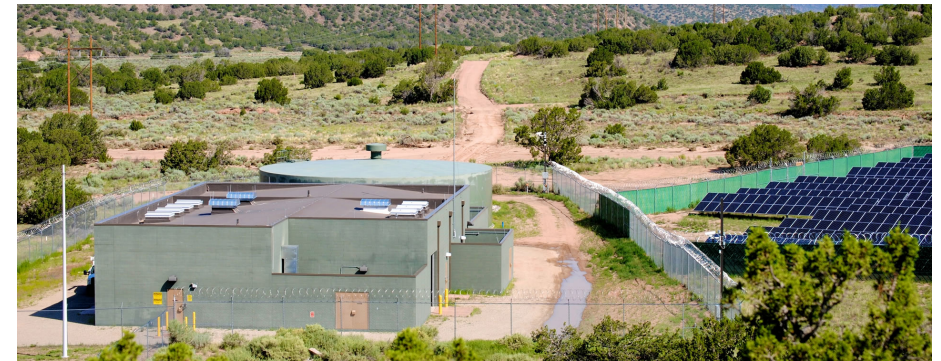
Buckman Direct Diversion – Santa Fe 1.5 MW solar to pump water 11 miles uphill from river to treatment plant (30% of energy)
