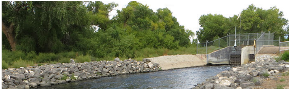
ABCWUA Southside WWTP - Albuquerque 4.5 MW (55Mgal/day) – 1.3 MW Solar, 1.2 MW Biogas
